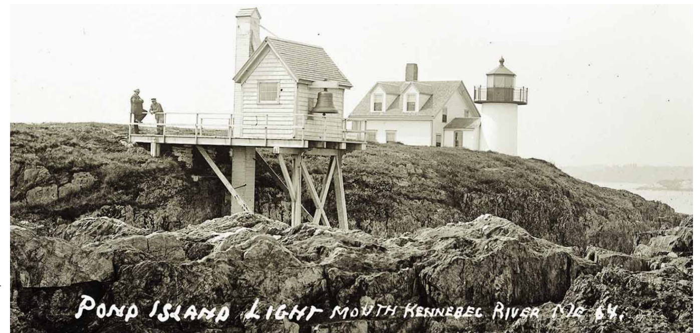
The two-ton bell functioned like a grandfather clock. Hand-winding a wheeled mechanism inside the shed activated a descending weight, releasing a heavy spring, triggering a sledgehammer to strike the bell.
