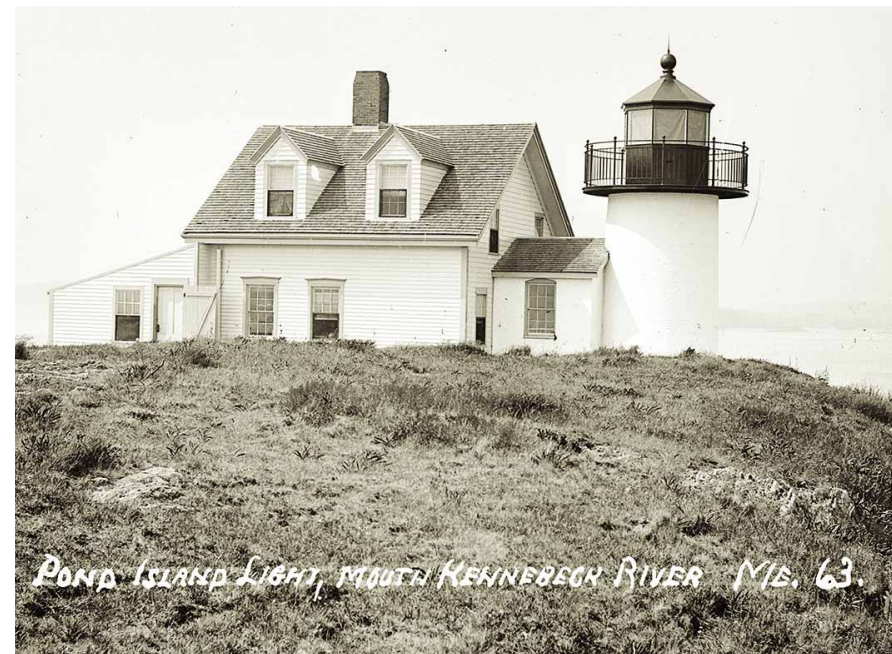
Winter storms often sent spray from crashing waves onto the leaky second-story windows of the Pond Island keeper's house. From November until April, Betty Brown kept a mop and pail in her upstairs bedroom.
