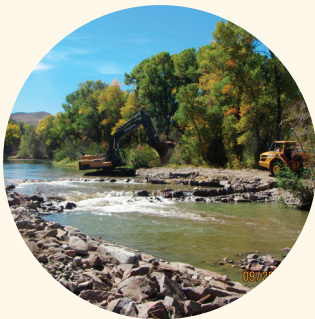
Constructed Riffle
