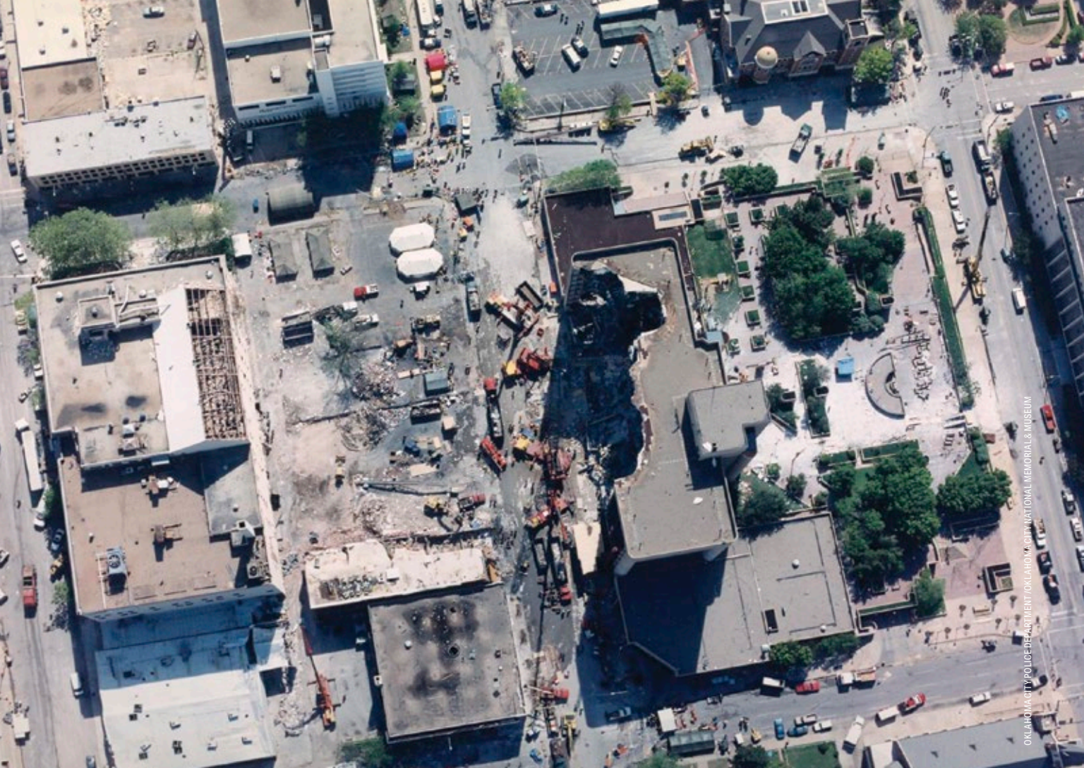
The Oklahoma City Police Department captured this aerial view of the Murrah Building shortly after the bombing.
