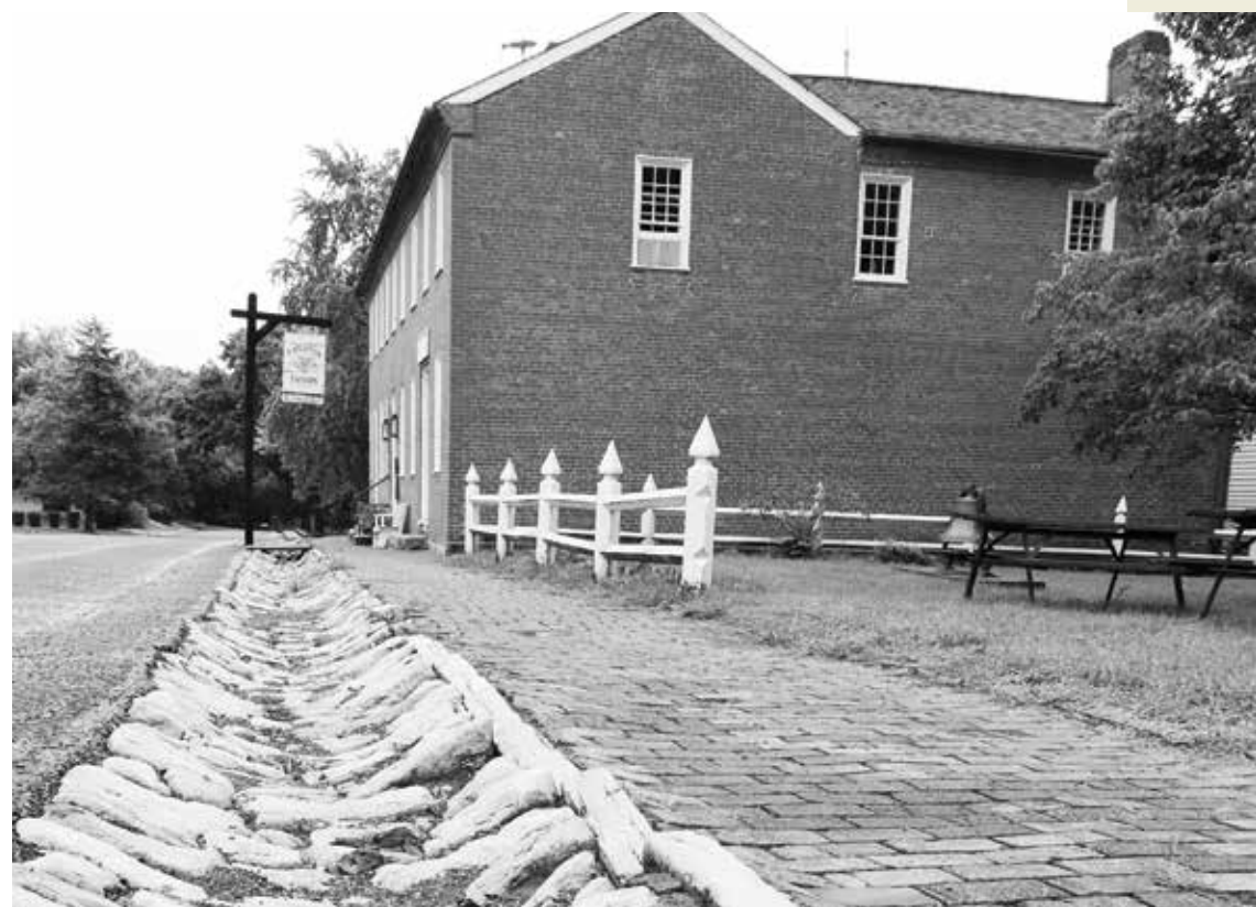
Horse and buggy was the common mode of transportation when enslaved laborers built these gutters in 1858. Today, the same stone gutters still carry storm water away from Main Street in 21st-century Arrow Rock.
