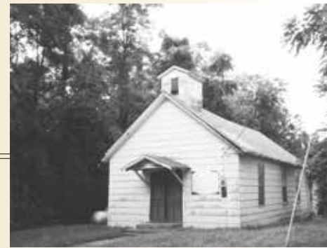
LEFT AND BELOW: Brown's Chapel Free Will Baptist Church held its last regular service in 1988 and sat unused for the next decade. The Friends of Arrow Rock began an extensive stabilization and restoration project on Brown's Chapel in 1998. The chapel is now available as an event and meeting space. The Friends also restored Brown's Lodge (not shown), which now houses the Arrow Rock Black History Museum.
