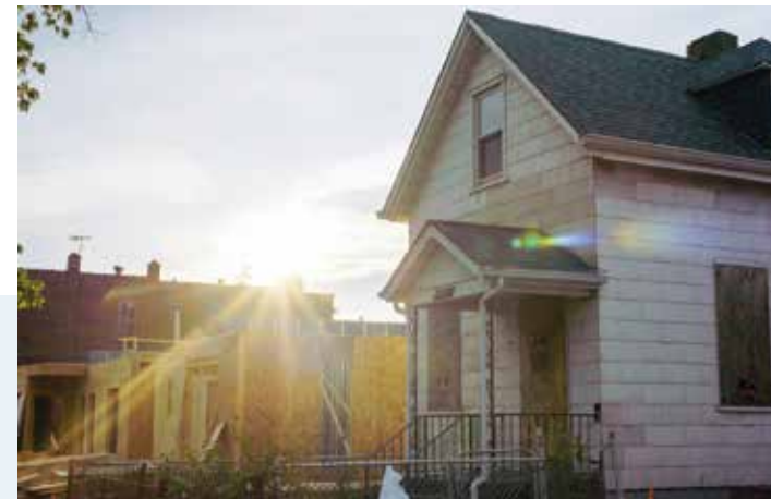
LEFT: In Forest Park Southeast, run-down houses are being torn down to make way for new or rehabbed projects. Once, the area was known more for its entertainment than housing. Now, the housing market is catching up.
