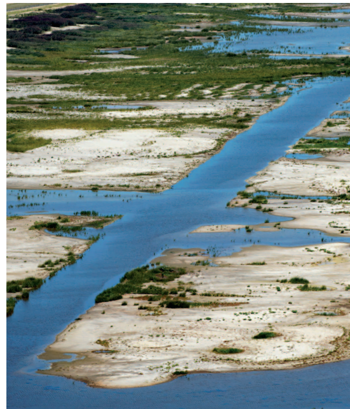
Seawater moves through man-made channels, carrying silt to help rebuild the marsh. Sand dug up during excavation of the channels was put along the banks.
