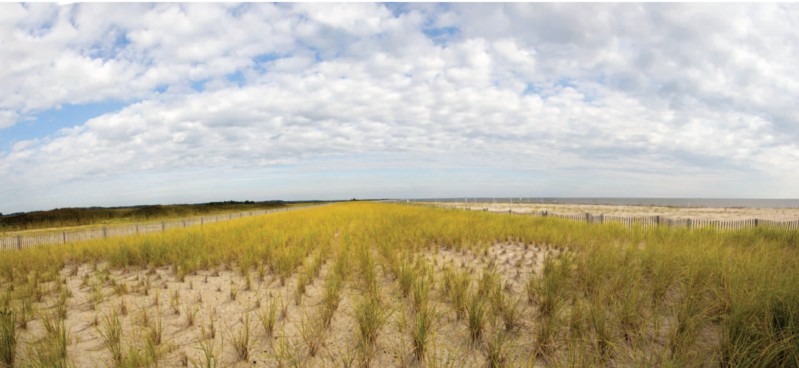
The top of the new 8,000-foot long dune at Prime Hook is planted in American beach grass to help hold the sand in place.
