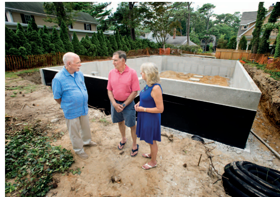
Attorney Gene Lawson, left, meets with clients Barry and Sharon Covington at their property in Rehoboth Beach. The Covingtons are fighting the city for the ability to include a backyard pool in the plans for their new home.
