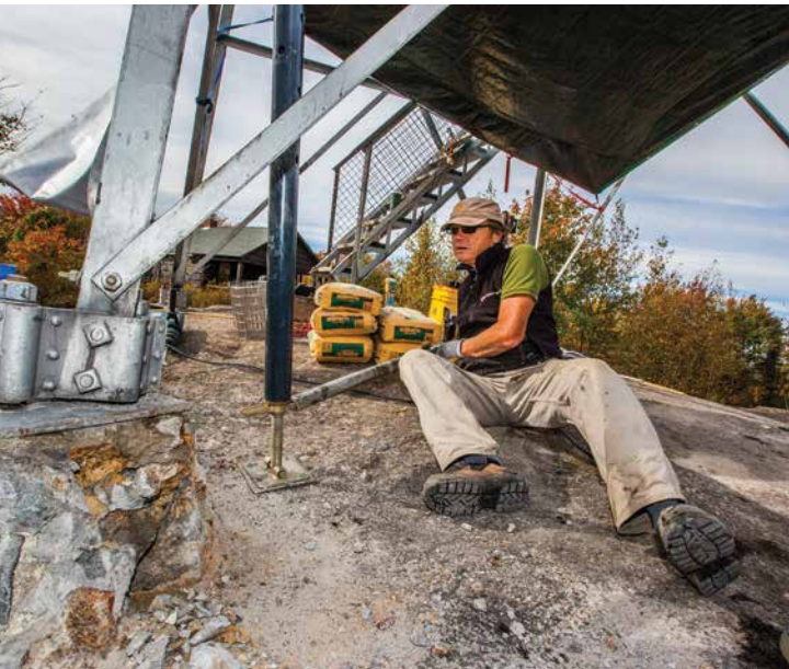
David Vana, of the fire-tower restoration company Davana LLC, replaces footers on Mount Arab's 98-year-old tower in Piercefild. From his 50-acre Bloomingdale property, below, Vana sells historic fire towers, but also custom, live-in lookouts based on 1935 U.S. Forest Service plans. Facing page: The autumnal view from Hurricane Mountain's fire tower.
