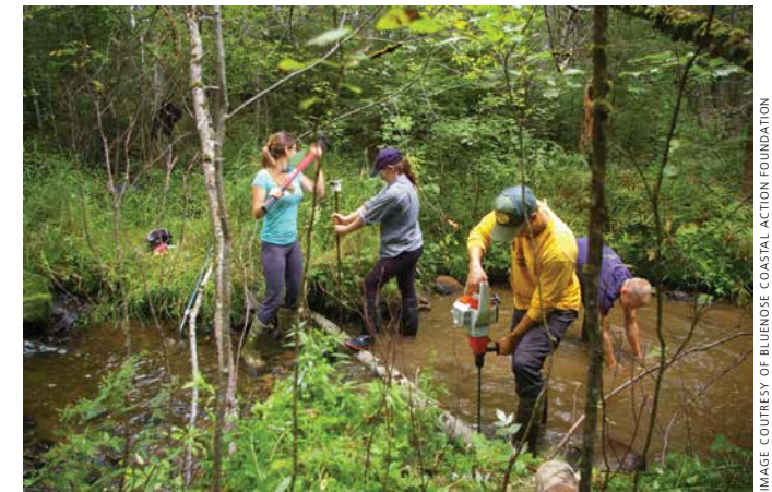
Staff of the Bluenose Coastal Action Foundation install a digger log as part of their stream restoration efforts.
