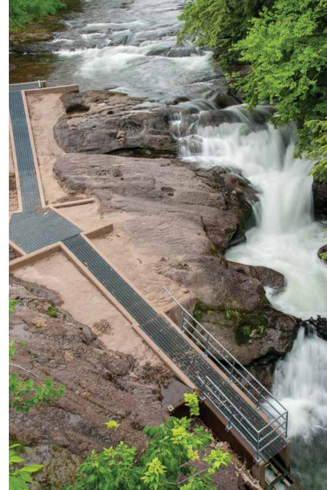
Left: Fish ladder circumventing barrier falls on the Waughs River allows salmon to swim further upstream. Above: Doug Bastow (left) and Edward Sampson of the North Colchester River Restoration Association.
