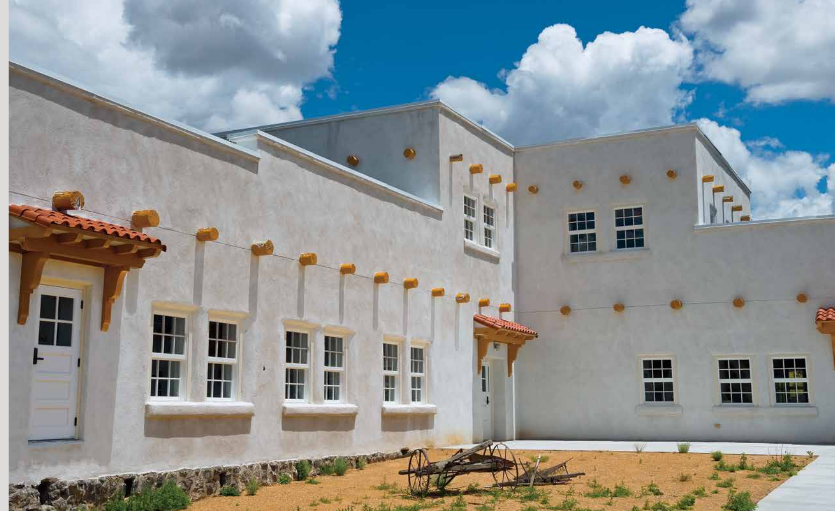
Built by WPA workers in the 1930s in the area's traditional style, the Sangre de Cristo Heritage Center is being revamped as a community center.
