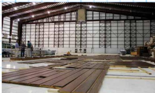
In a hangar at the Northwest Arkansas Regional Airport, workers laid out an exploded view of the house from which they could pull lumber and fixtures.
