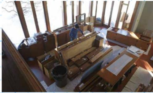
The work started inside the home, where the interior fixtures and mahogany board and batten were removed, inventoried and carefully packaged, piece by piece.
